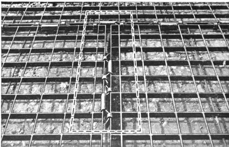
Figure 97. Joint in bar-and-rod mat with crimping completed.
